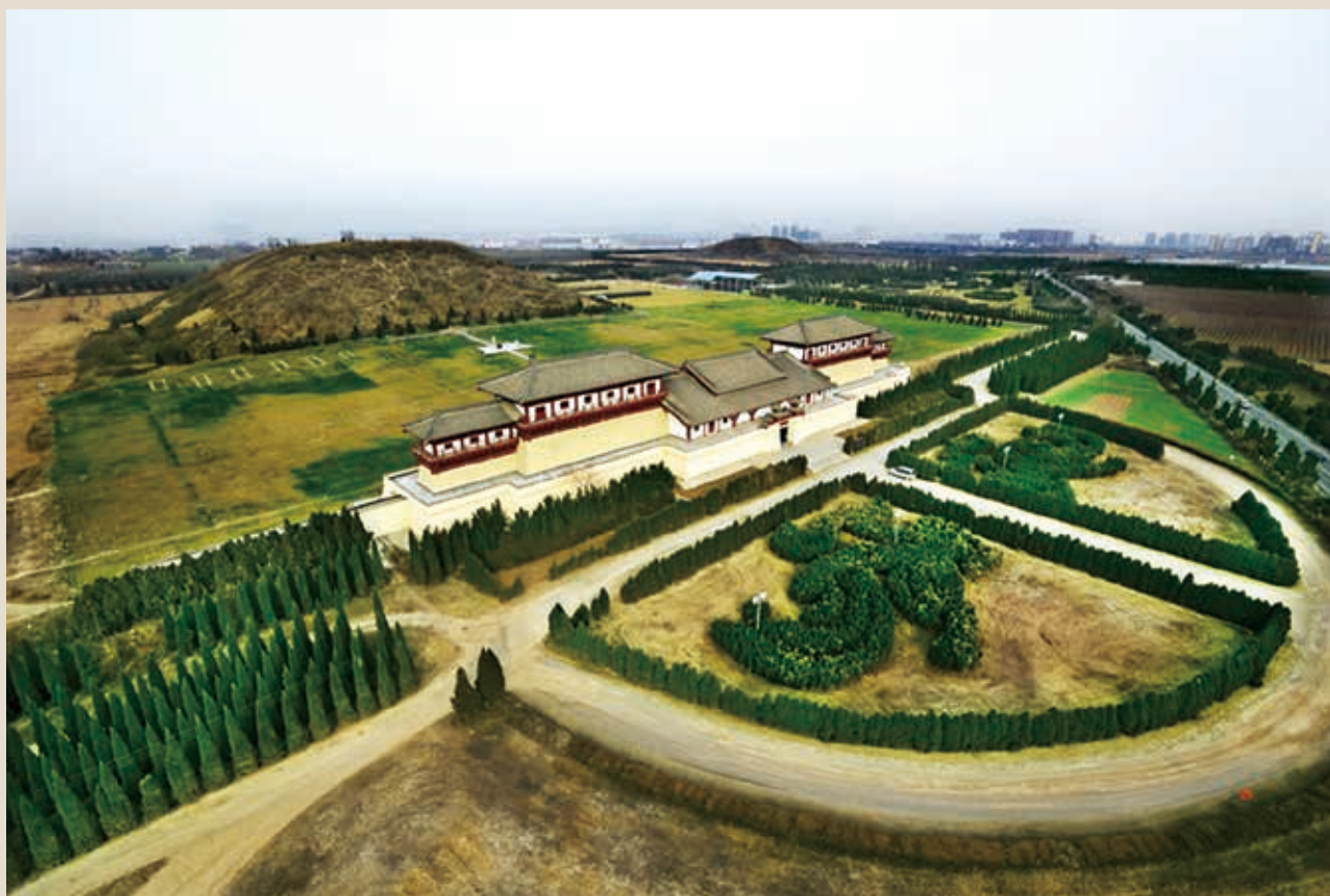
帝陵南阙门遗址保护展示厅 The Exhibition Hall of the South-Gate Tower
